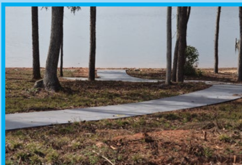
CONCRETE CART PATH
