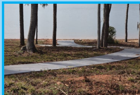
CONCRETE CART PATH
