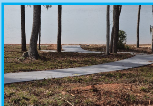
CONCRETE CART PATH
